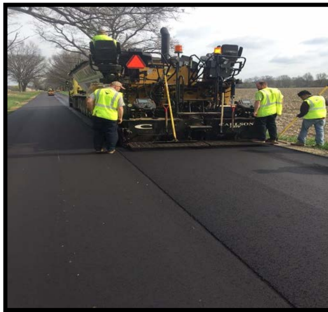
28th Street – HMA Wedging, Chip Seal and Fog Seal, Brady Township
